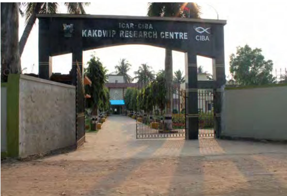
Renovation of boundary wall to safeguard the property at KRC of CIBA at Kakdwip
