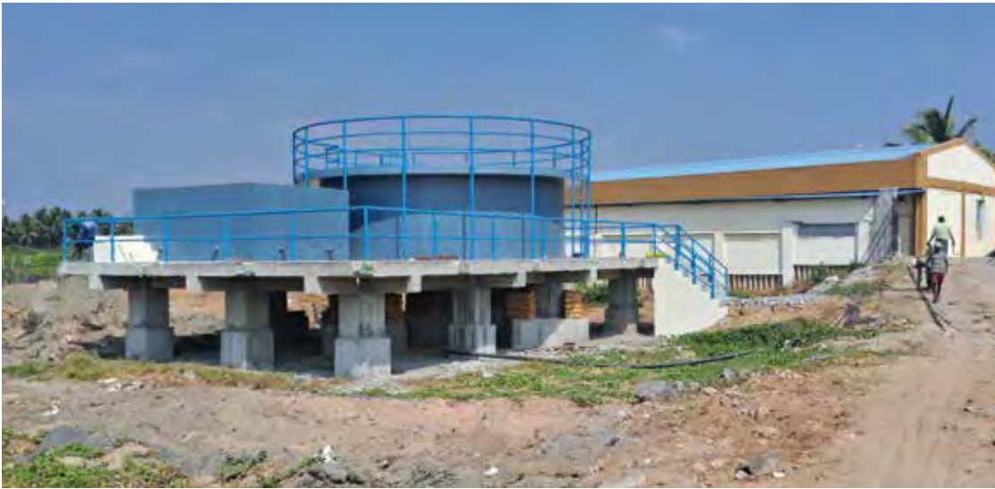
Construction 25 ton RCC tank in Fish hatchery at MES of CIBA
