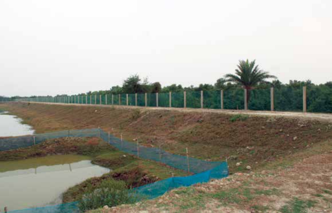
Renovation of main dyke at KRC of CIBA at Kakdwip
