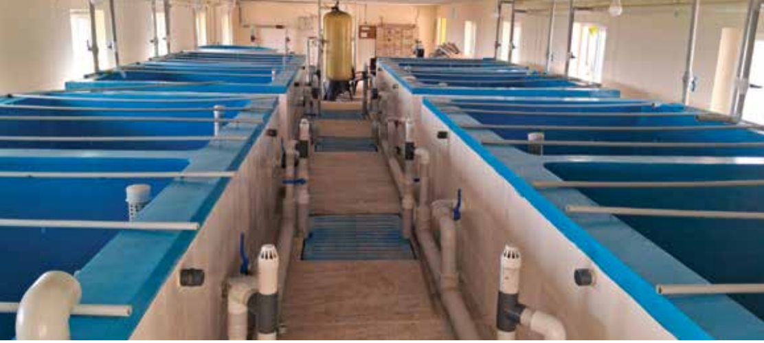
Renovation of seed bank shed at MES of CIBA
