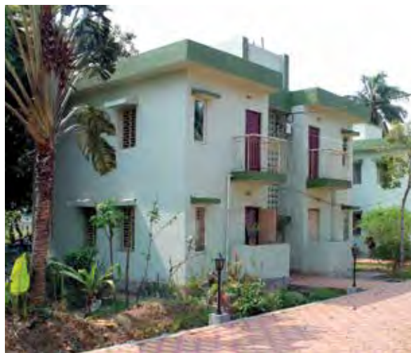
Renovation of staff Quarters type- 1,2&3 at KRC of CIBA at Kakdwip
