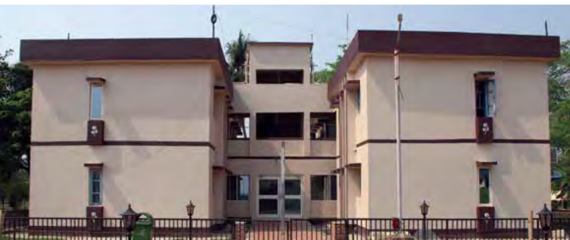
Renovation of staff Quarters type- 1,2&3 at KRC of CIBA at Kakdwip
