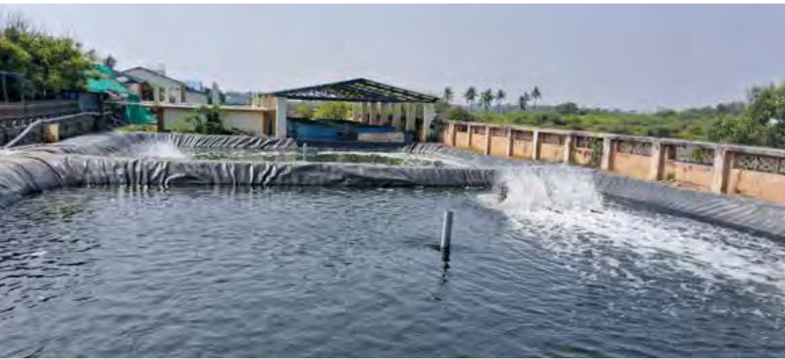
Renovation brood stock pond at CCD hatchery at MES of CIBA
