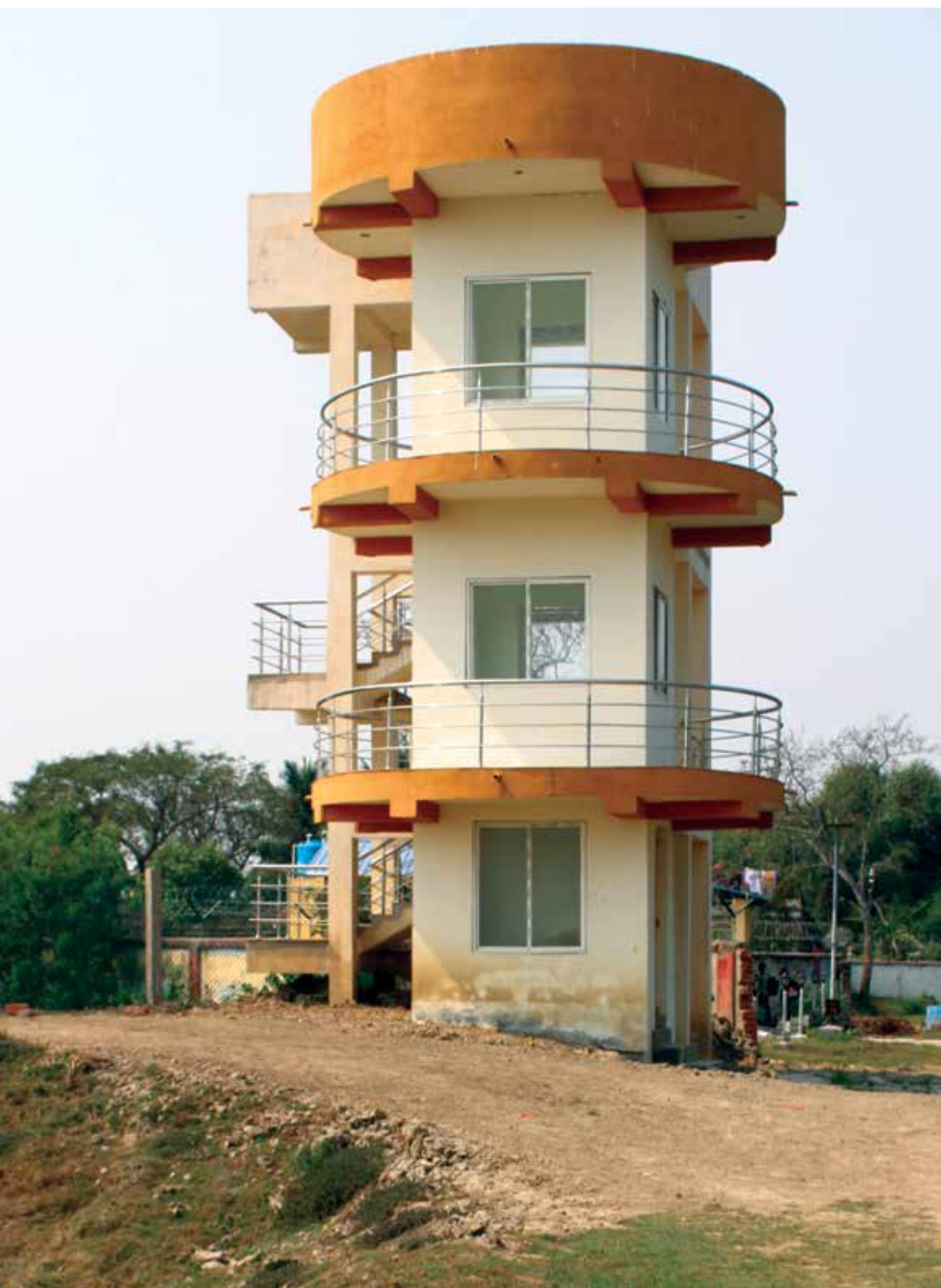
Renovation security cabin at KRC of CIBA at Kakdwip
